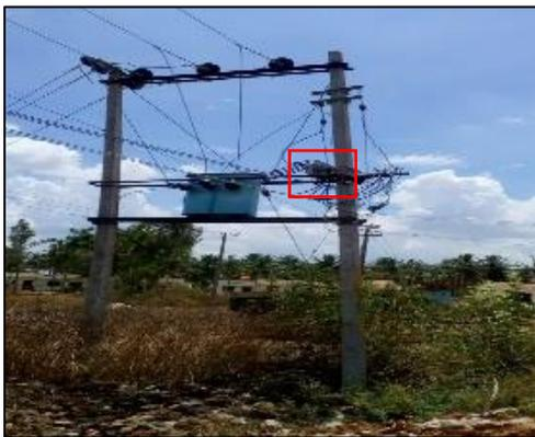
Figure 6: Meter placed high
