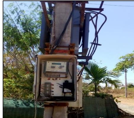
Figure 5: Meter not connected
