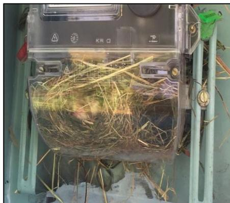
Figure 8: Bird's nest inside the newly installed DT meter
